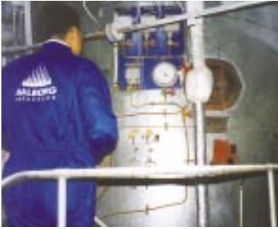
Commissioning of boiler.
