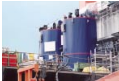
2 x MISSION™ OL boilers installed in Korea.
